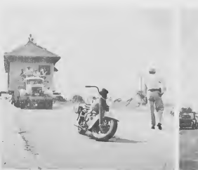
CLEARING THE way for this section of the former Lago office building is a government motorcycle policeman. The movers were preparing to cross the Spanish Lagoon Bridge. PREPARANDO CAMINA pa e seccion aki di e anterior oficina di Lago ta un pulis di gobierno ariba motorcycle. Aki nan ta preparando pa cruza Spaans Lagoon.
